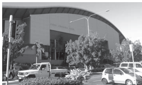
Cairns Convention Centreの外観
